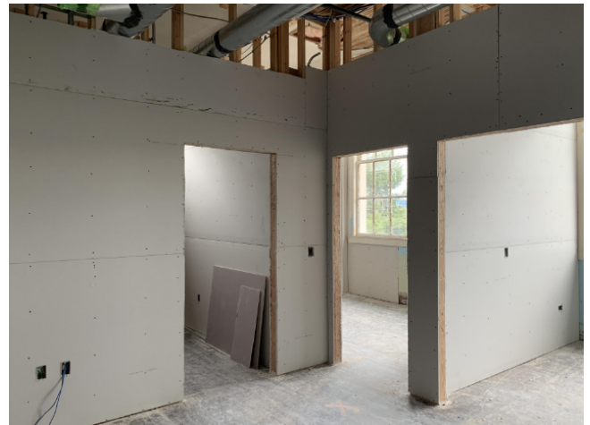
Level Two Drywall Installation
